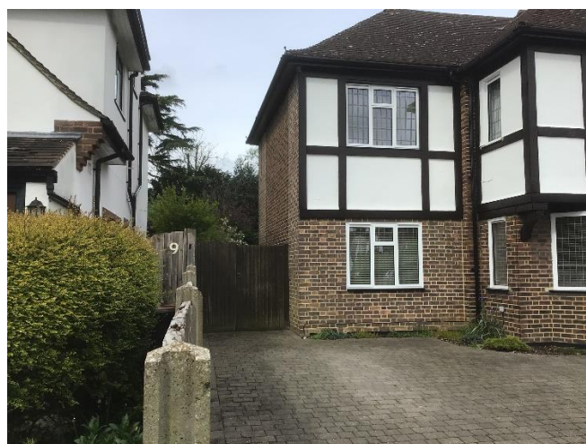
Figure 14: Existing side space between the host dwelling & No. 11 The Meadow
